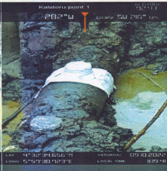
PICTURE 2: SHOWING POINT A AFTER REPAIRS
