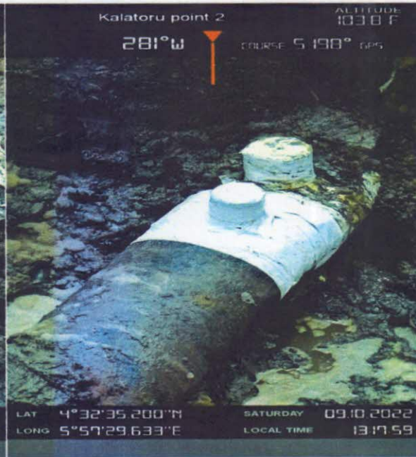
PICTURE 4: SHOWING POINT B AFTER REPAIRS
