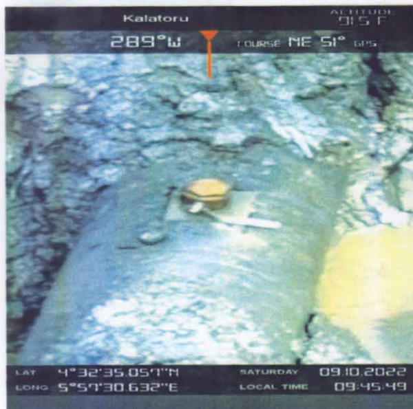
PICTURE 1: SHOWING INSTALLED 3" VALVE AT POINT A.
